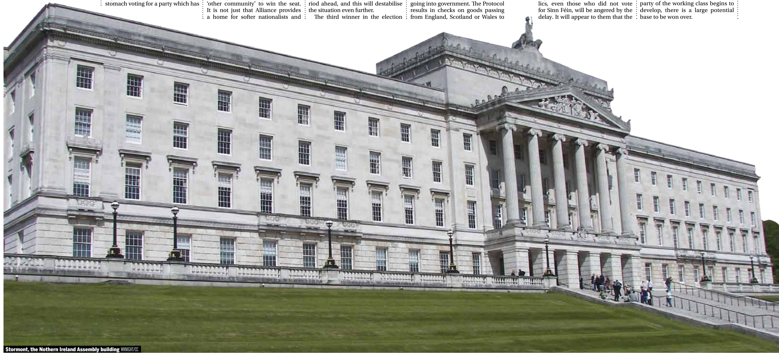
Stormont, the Northern Ireland Assembly building WRIGHT/CC
